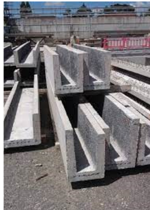
U-shaped precast beams Source: Park and bull, 1986
