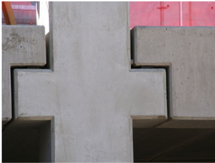
Precast beam-column connection using corbel
