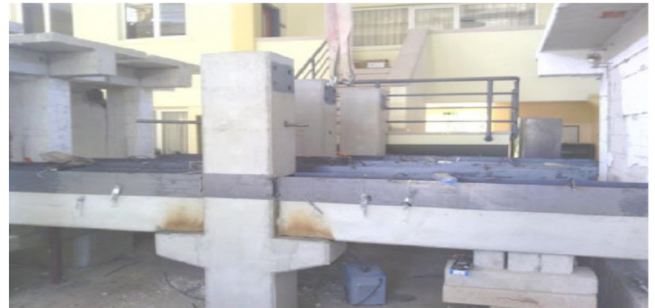
Precast joint with emulative-welding technique
